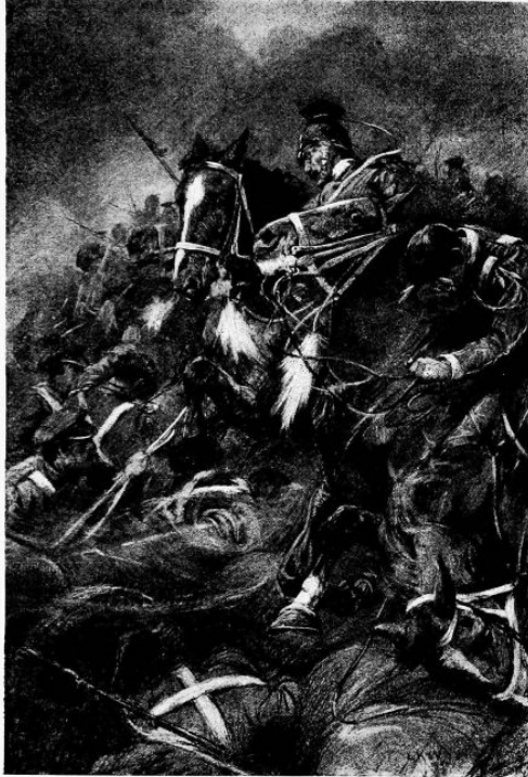
"The batteries are reached and carried."
